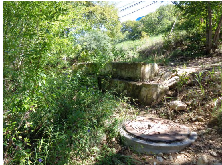
Photopoint: 40 Direction: N Manhole cover, armored wall and both Japanese and Chinese privet are found at this location.
