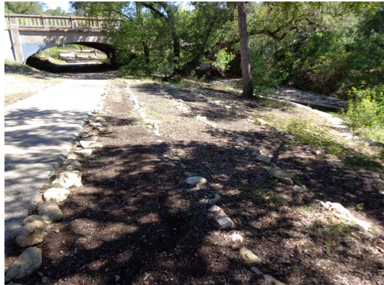
Photopoint: 26 Direction: NNE Rock terraces are slowing soil erosion, but this area has yet to revegetate.
